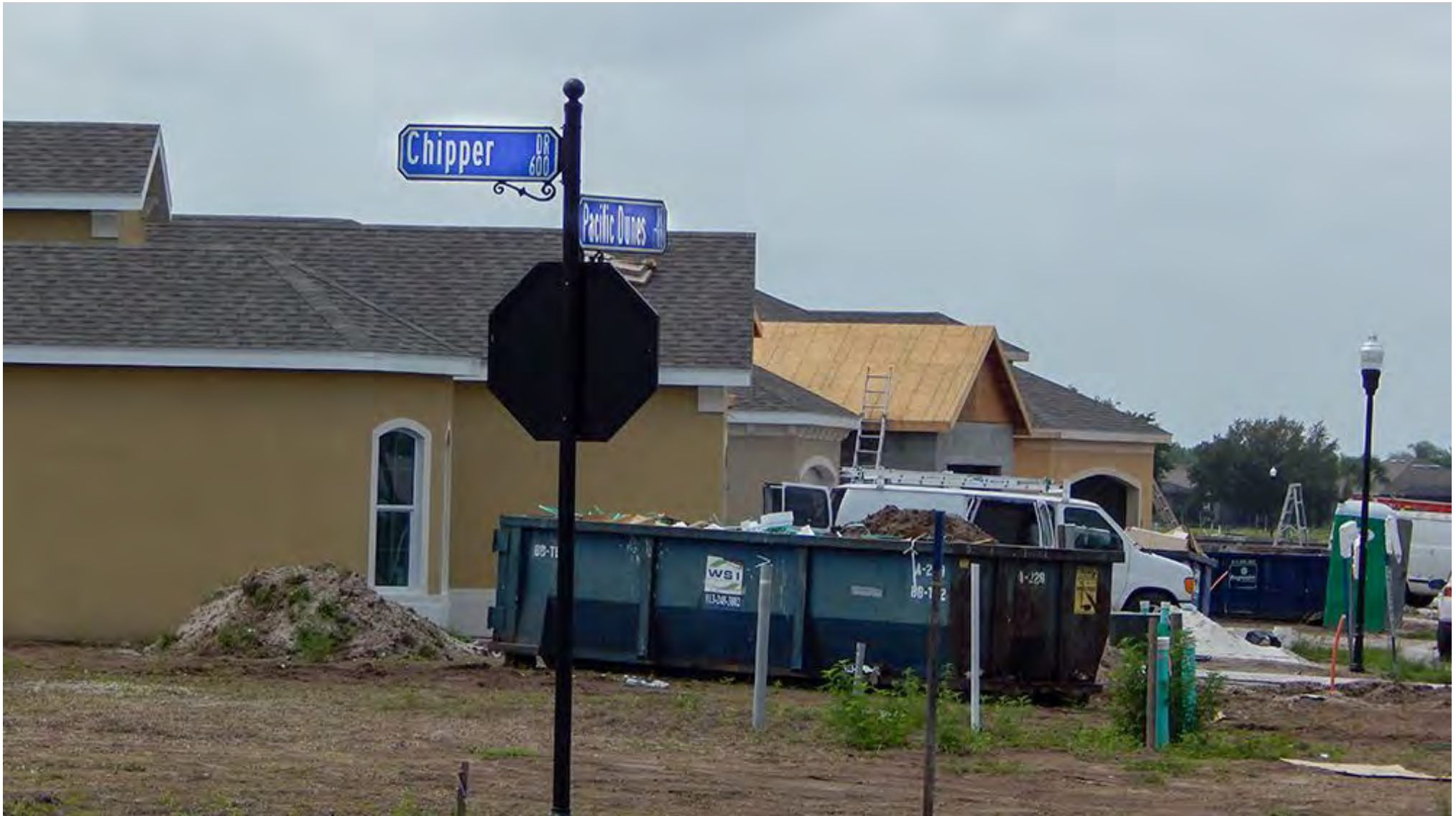
Single-Family Homes Being Built
