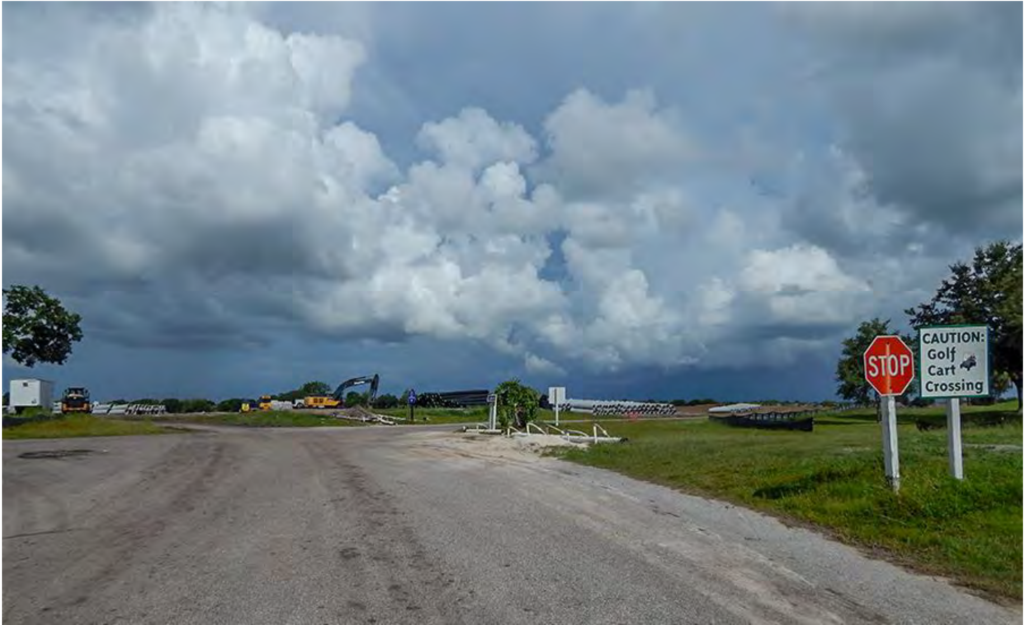
Infrastructure Work in Progress
