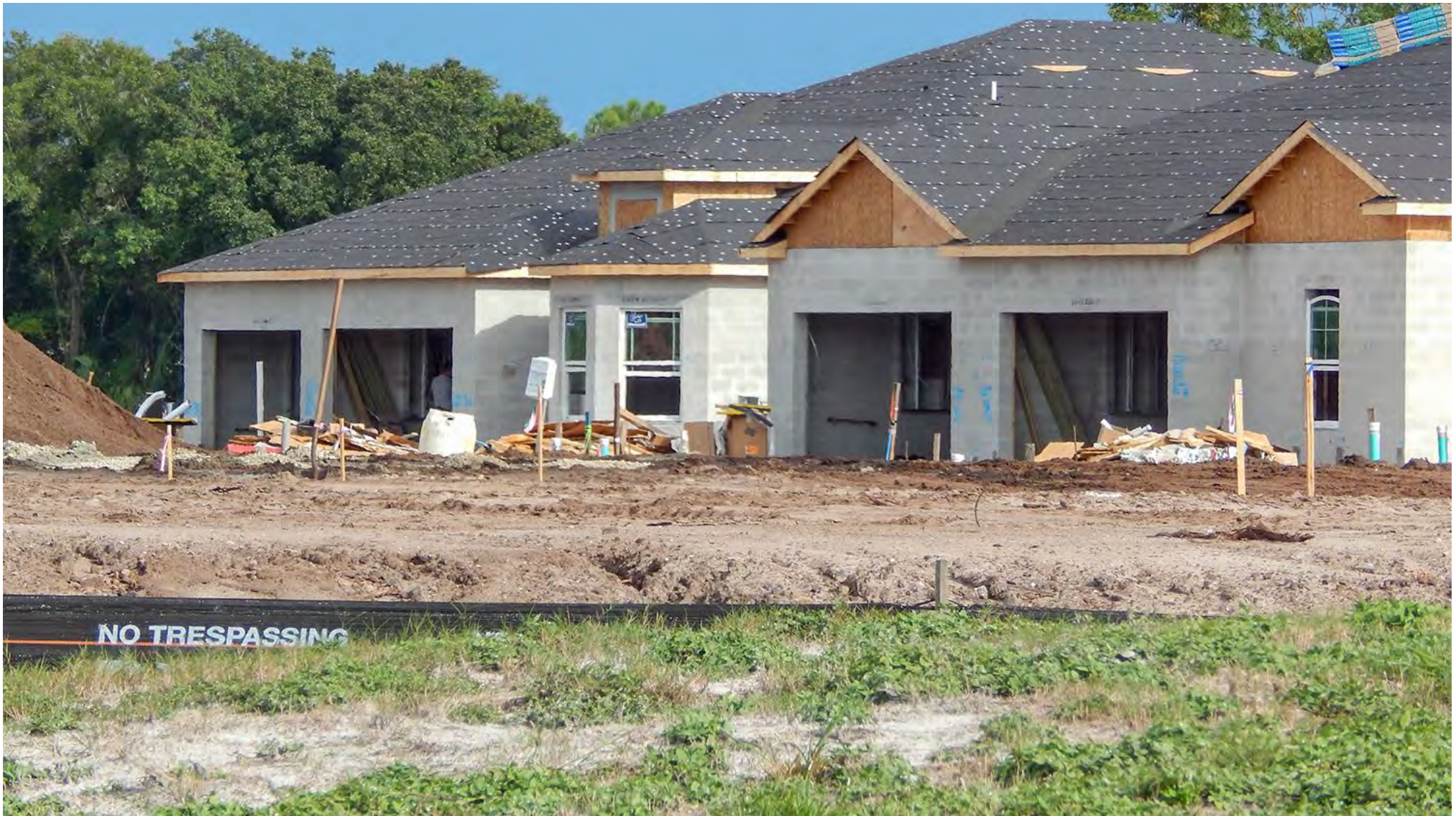
Twin Villa Models Under Construction
